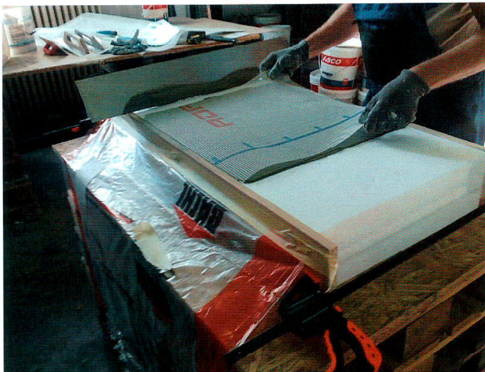
- application of reinforced base coat of ETICS -
