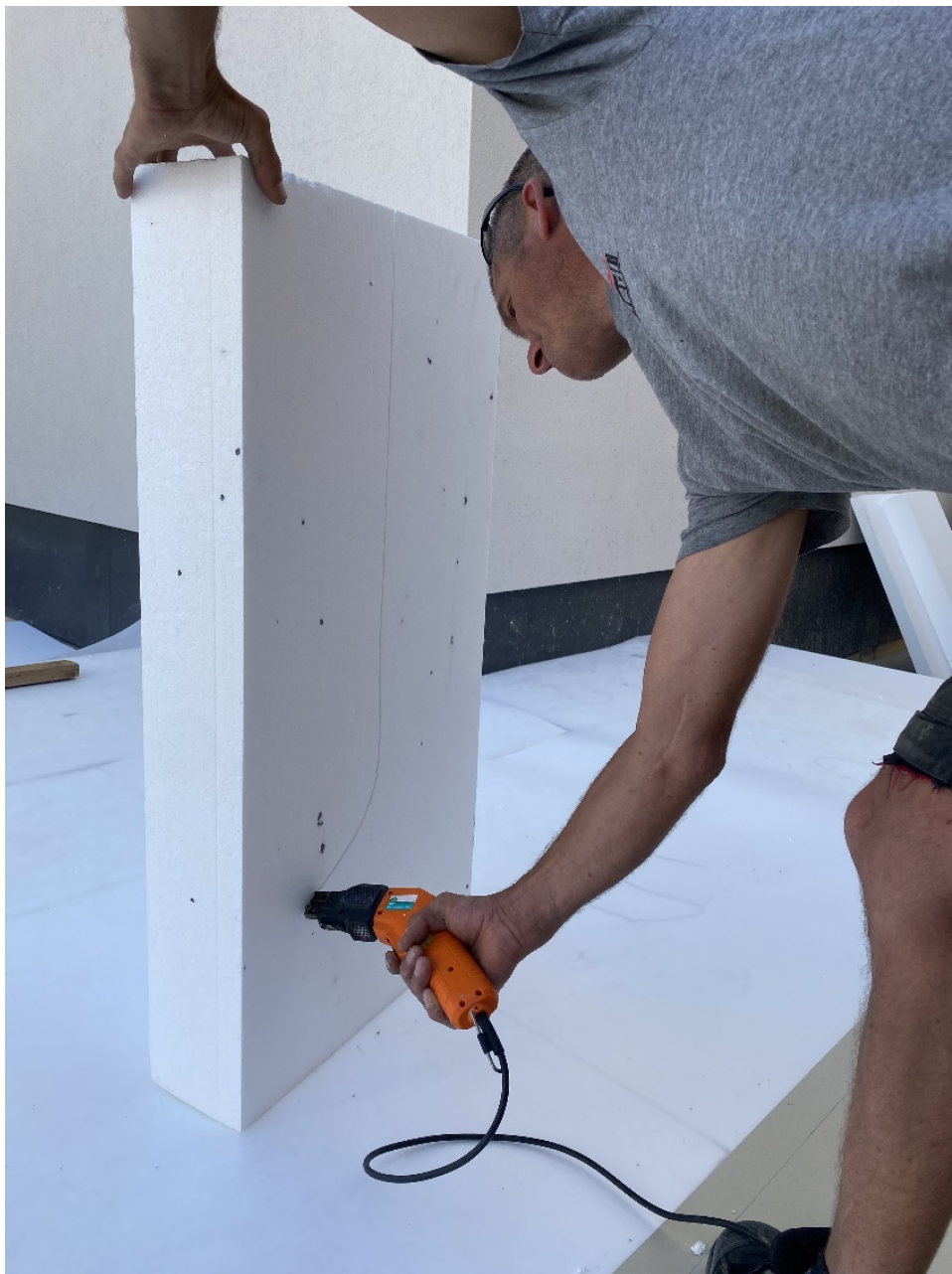
Figure 4. Worker using a hot wire to cut EPS (source: IVH, EUMEPS, NEPSA and EPS-branchen).
