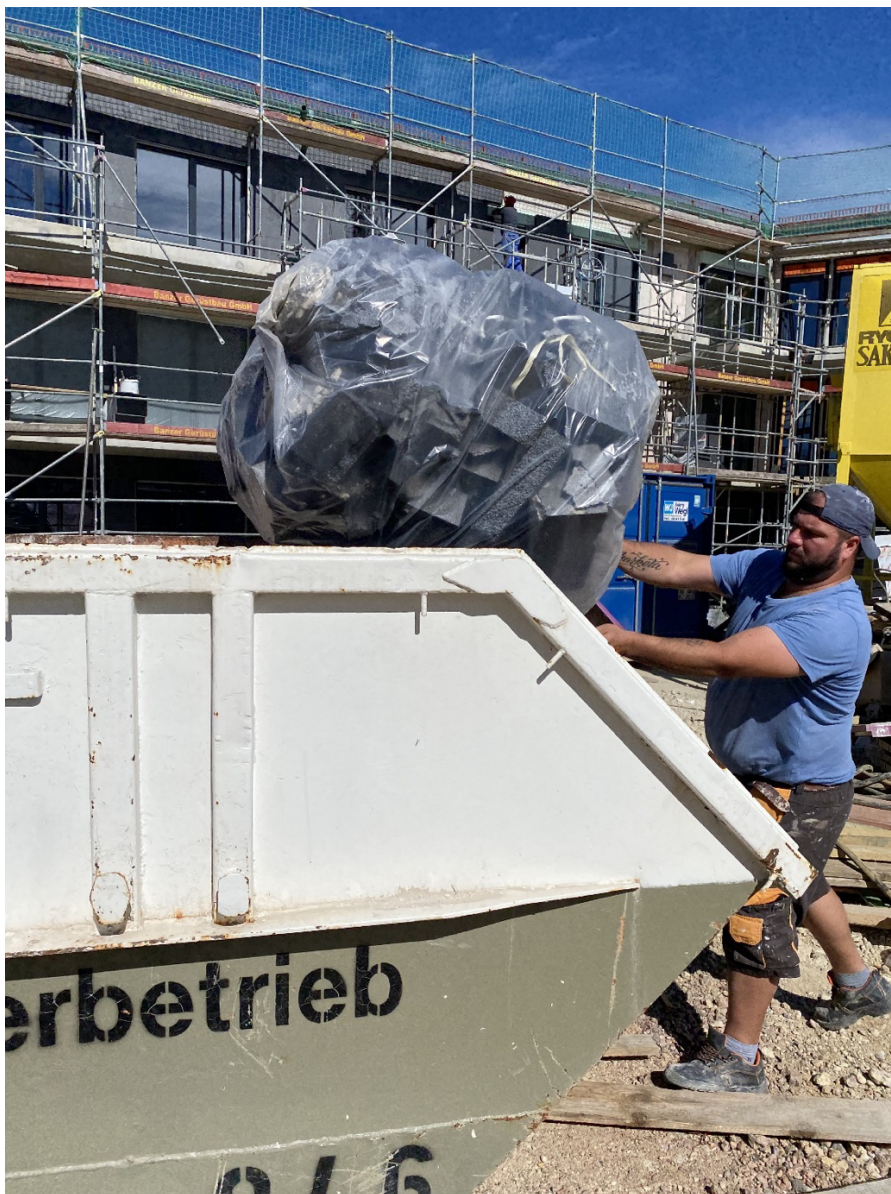
Figure 5A. Correct sorting of EPS waste (source: IVH, EUMEPS, NEPSA and EPS-branchen).
