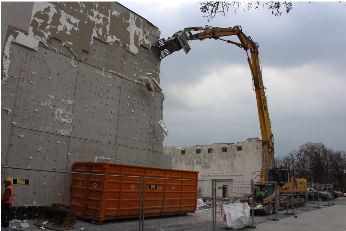
Figure 6. Example of EPS/XPS demolition waste sorting (source: IVH, EUMEPS, NEPSA and EPS-branchen).
